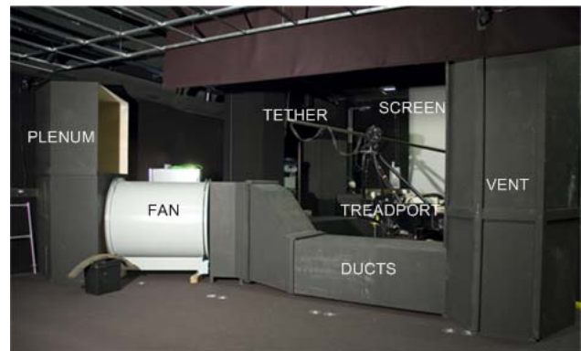
Figure 11 Full-scale TreadPort Active Wind Tunnel while under construction.
